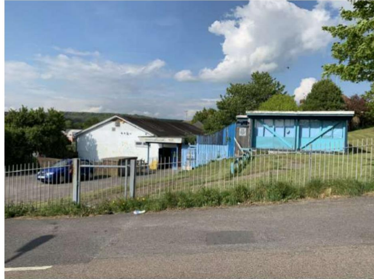
Site view of northern corner of Hodshrove Lane & Hodshrove Rd.
