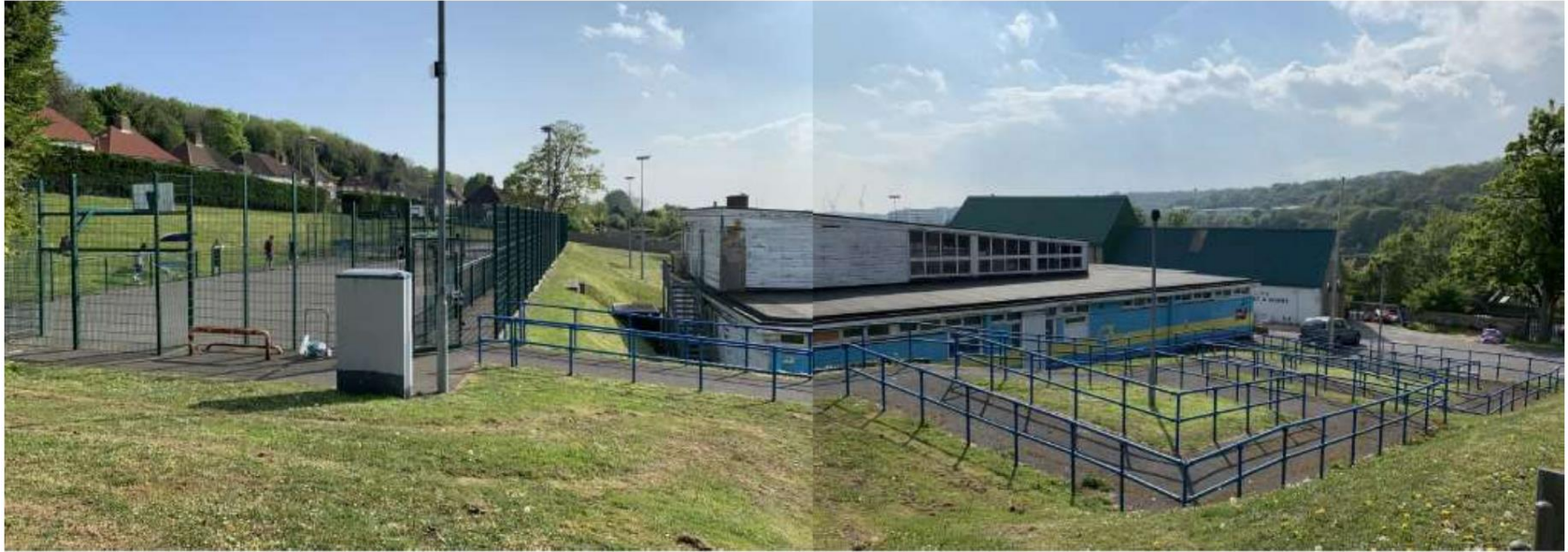
View showing the 67 Centre and ramps up the steep slope.
